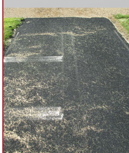
Figure 10 - Faded track runway stripe
