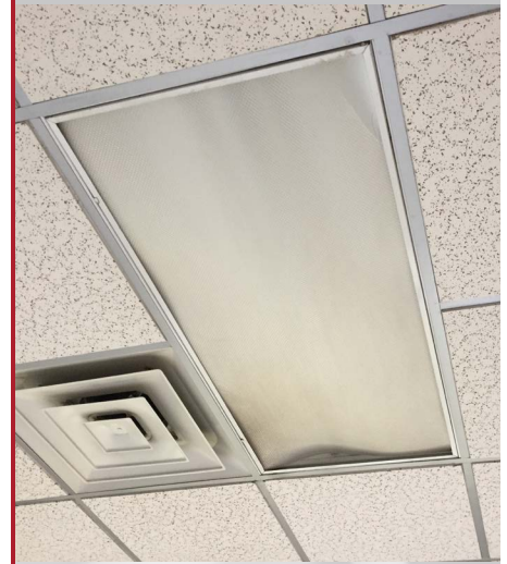
Figure 8 - Light fixture with warped lens
