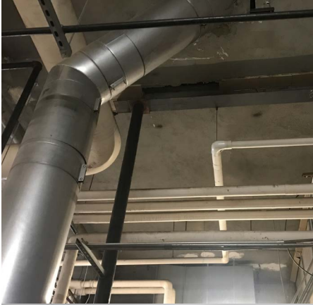
Figure 1 - Beam in boiler room
