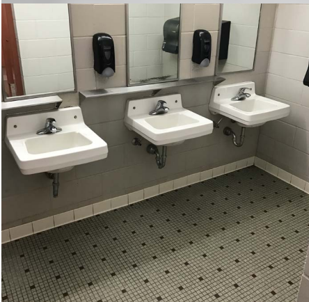
Figure 2 - Glazed block walls and tile floors in restroom
