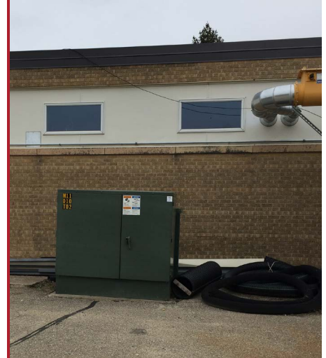
Figure 1 - Ground-mounted transformer
