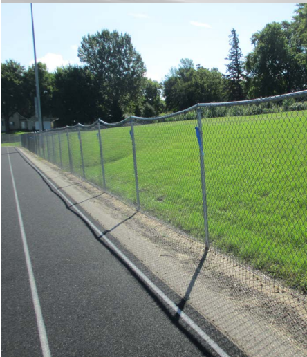
Figure 8 - Sagging fence near track
