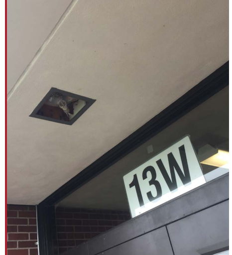
Figure 7 - Light with broken lens
