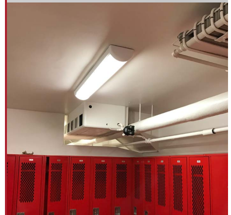
Figure 12 - Exhaust air missing in concession stand
