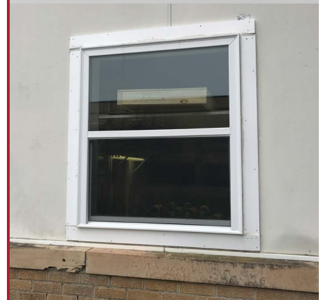
Figure 6 - Vinyl windows in shop space
