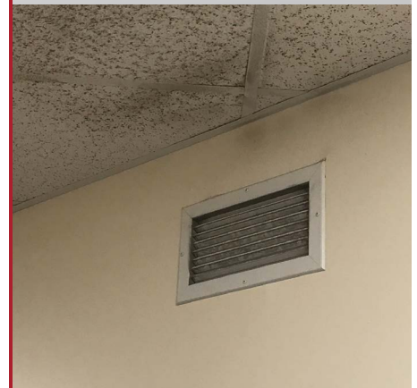
Figure 20 - Transfer grill for kitchen
