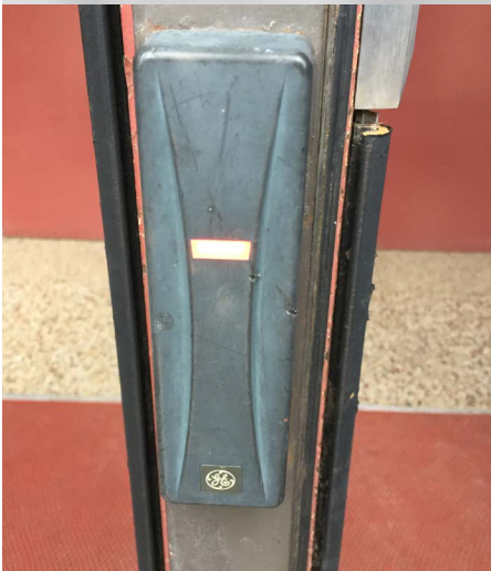
Figure 2 - Typical access control card reader
