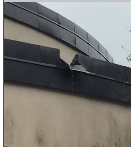
Figure 5 - Close up of EFIS surface
