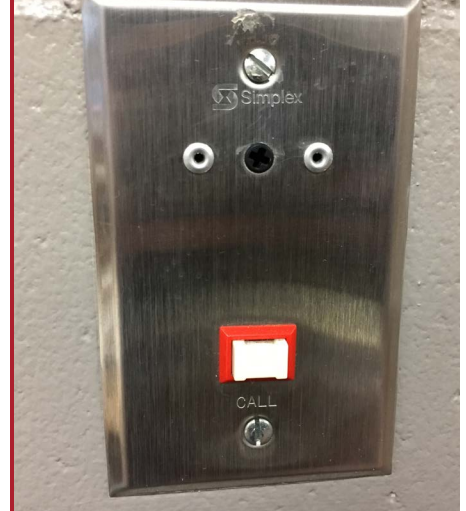
Figure 3 - Typical intercom call button
