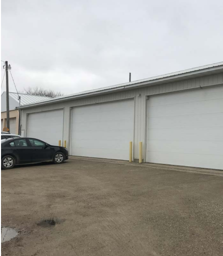
Figure 4 - Overall view of bus garage
