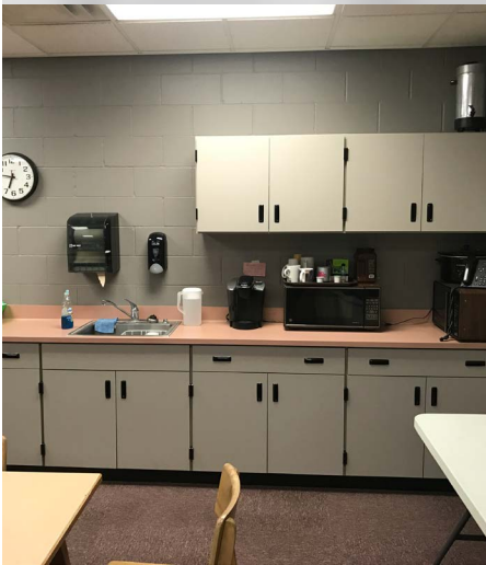
Figure 2 - Typical classroom sink which is not ADA compliant
