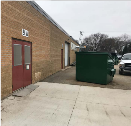
Figure 3 - Receiving room/janitor space, which lacks a dock
