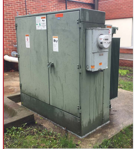
Figure 1 - Ground-mounted transformer
