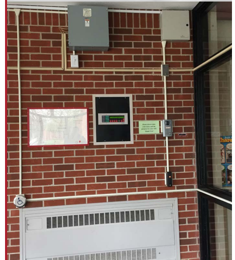
Figure 3 - Existing secured entrance
