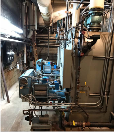
Figure 1 - Two existing steam boilers
