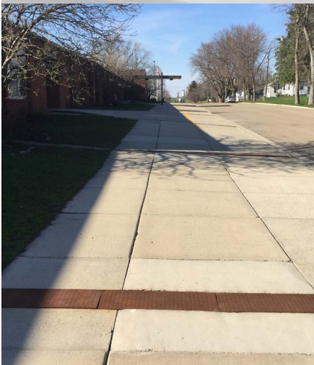
Figure 9 - Warped grates
