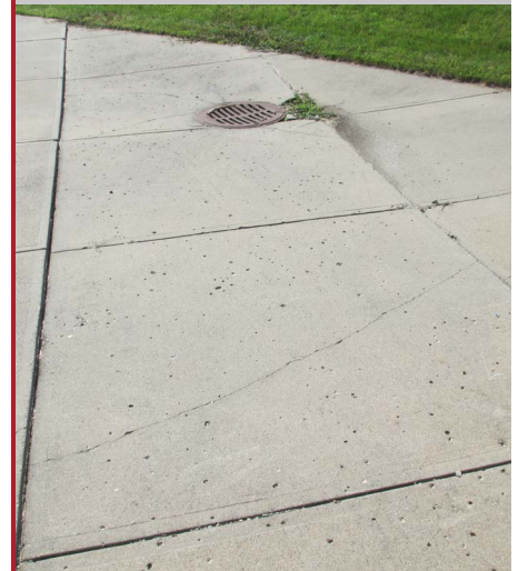
Figure 5 - Catchbasin in shop area
