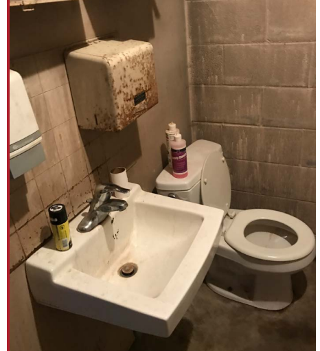
Figure 1 - Bus garage restroom
