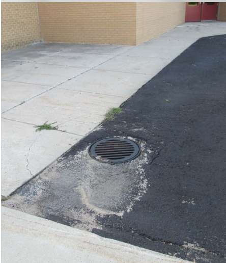
Figure 2 - Catchbasin in north staff lot
