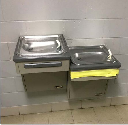
Figure 4 - Broken electric water cooler
